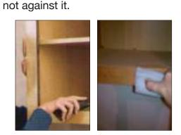
• Use a sanding block with 150 grit paper to sand in one direction (INWARD), to smooth the
